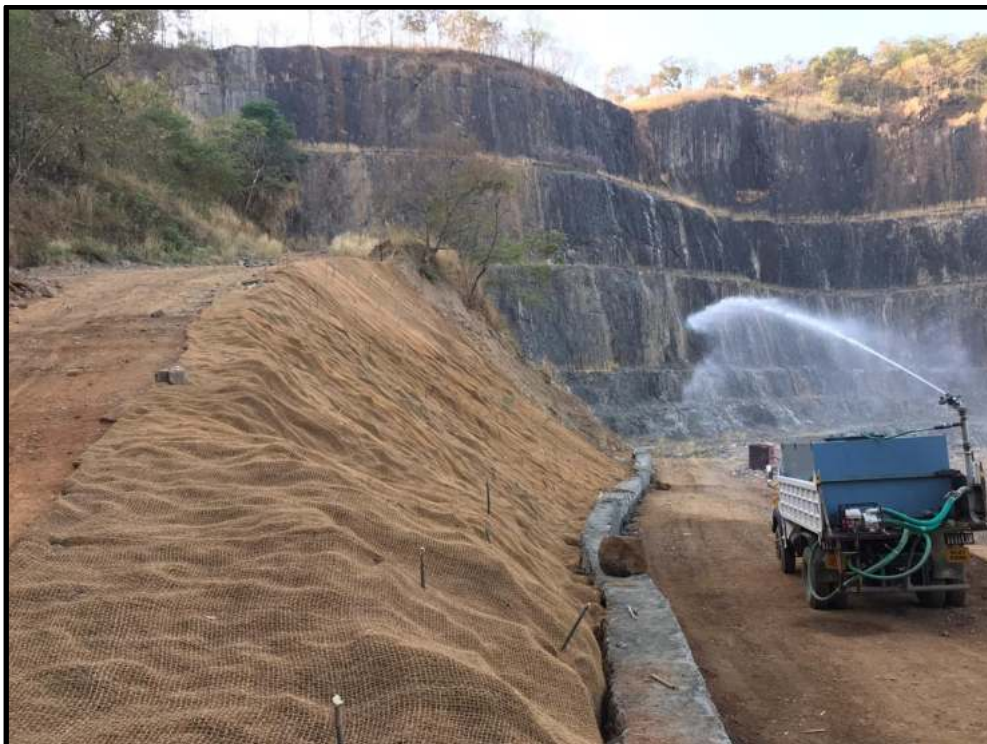
Photograph showing the Sprinkler system installed in crusher plant and tipper lorry
